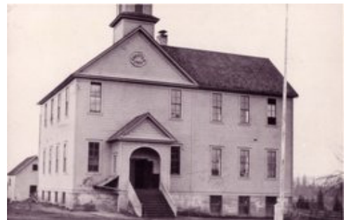
Old school after being raised up to add floors.
